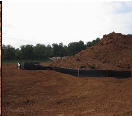
Correctly Installed Stockpile Protection
