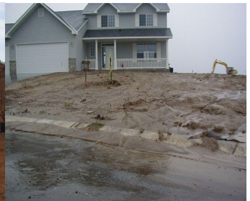
What Happens Without Appropriate Erosion and Sediment Control
