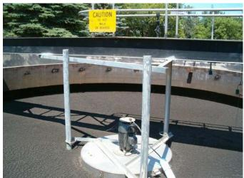
Waste activated sludge (WAS) is stored in the WAS holding tank ahead of thickening. The WAS holding tank was an existing gravity thickener in the previous plant process layout. The WAS holding tank has been retrofitted to provide at least five days of WAS storage so the thickening process can be flexible. A floating mixer is used to mix the contents of the tank.
