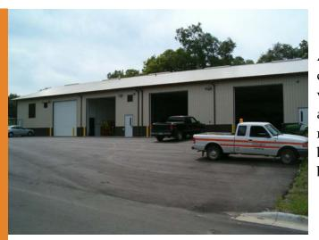
A new Maintenance Garage was constructed on the WWTP site to provide vehicle, equipment and parts storage, and to provide area for WWTP maintenance procedures. The new building is a wood-framed metal building with several overhead doors.
