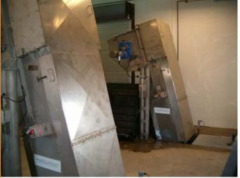
As the wastewater enters the Fairmont WWTP the first treatment step is screening. Two mechanically cleaned bar screens remove sticks, rags, large solids and other debris that may prove harmful to downstream plant equipment. Following screening, the influent flow is sampled for influent characteristics and measured thru a Parshall flume.
