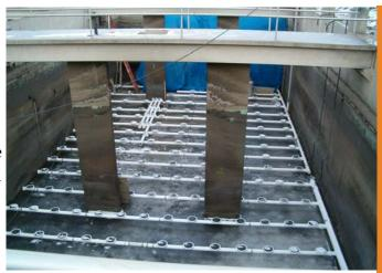
microorganisms to consume the organic material in the wastewater. The fine bubble diffused aeration system includes flexible membrane diffusers to efficiently transfer oxygen to the microorganisms.
