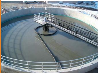
Two new 75-foot diameter primary clarifier tanks are used to settle the wastewater and separate the liquid from the solids by gravity settling of solid particles. The primary clarifiers also serve the main function of phosphorus removal. Ferric chloride is added to each of the primary clarifiers to chemically bind the phosphorus molecules and precipitate out the phosphorus as solids.
