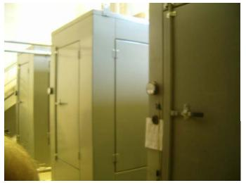
The aeration air supplied to the aeration tanks is from three 125 Hp positive displacement blowers. The blowers are energy-efficiently controlled to supply a preset airflow to maintain a target dissolved oxygen level in the tanks. The new aeration blowers are enclosed units to reduce noise levels in the blower room. The new blowers are located in the existing WWTP blower room.
