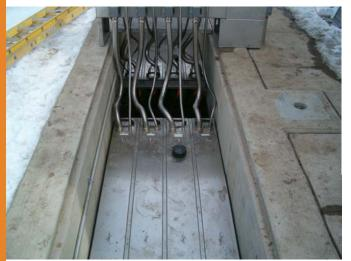
The secondary clarifier effluent is sent to the ultraviolet (UV) disinfection system for final disinfection before final sampling and discharge to Center Creek. The low pressure, high intensity lamps inactivate any bacteria that would be discharged.
