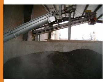
A covered biosolids storage area is adjacent to the Solids Processing Building. The storage area provides enough biosolids storage in one of two cells for a minimum of 180 days of biosolids storage. The metal canopy cover has been provided to keep any precipitation from mixing with the dried or dewatered biosolids products. Prior to spring planting or after fall harvest the stored biosolids will be removed and land applied to area farmland to use for its fertilizer value.
