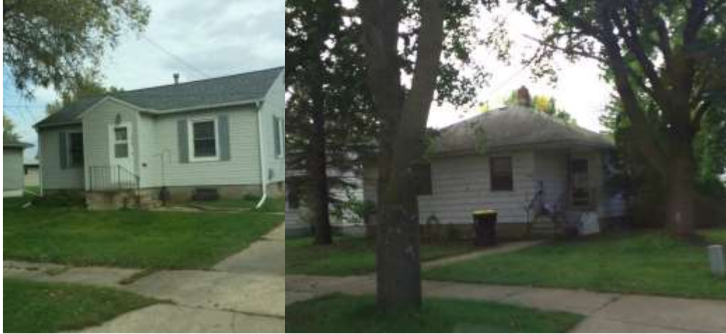
Image 5: These two photos show the difference between former worker housing in northern Fairmont that have been rehabilitated to the left, and slightly distressed to the right.
