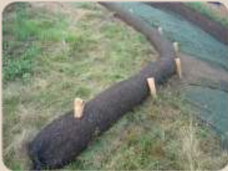
A sediment control log, such as the one shown above, captures dirt and debris before it washes away. Photo by Washington Conservation District.
