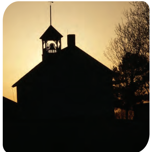
CHAPEL BELL TOWER AT HERITAGE ACRES
