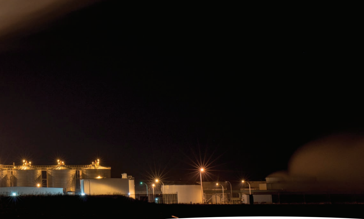
ABOVE: VALERO PROCESSING FACILITY IN FAIRMONT OPERATES 24/7, CRUSHING APPROXIMATELY 110,000 BUSHEL OF SOYBEANS DAILY.
