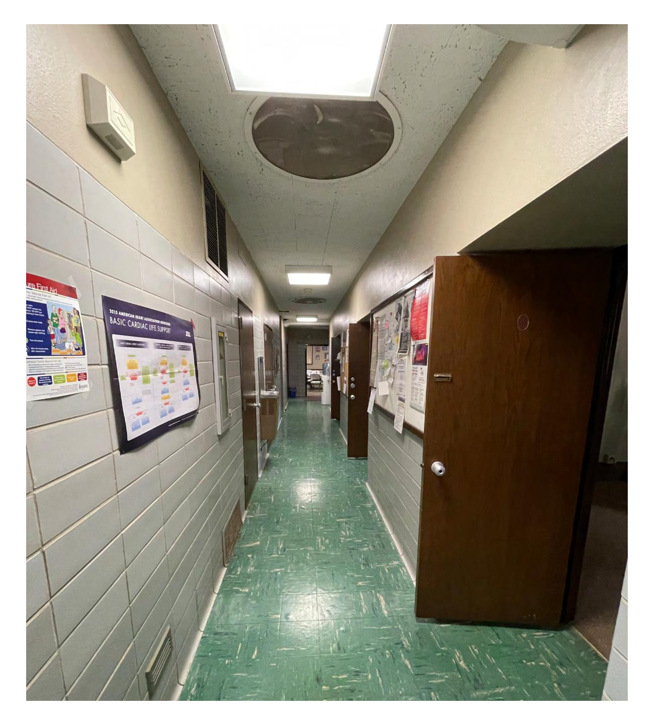
• interior lacks natural light; old skylights in the corridor were removed & covered due to leaking
