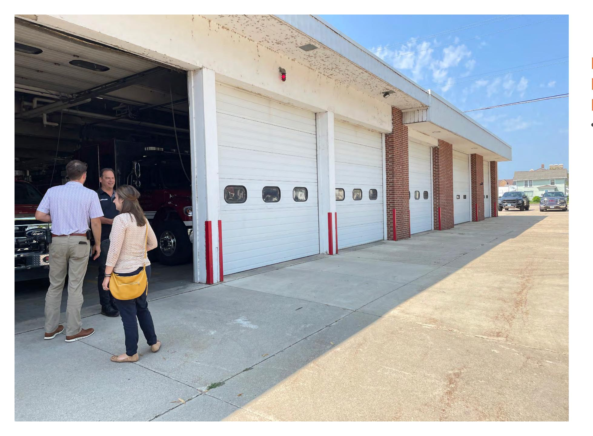
paint peeling on fascia & soffit; apparatus bay doors are too narrow and short for new apparatus
