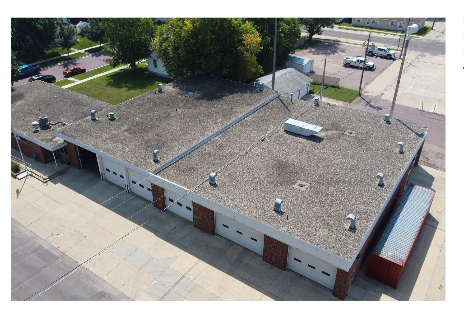
dated roof and limited roof drains cause roof leaks when it rains and when the snow melts
