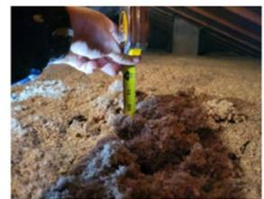
Image of an under-insulated attic in Comfrey. The recommended level of R49 insulation is about 16 inches of continuous insulation.
