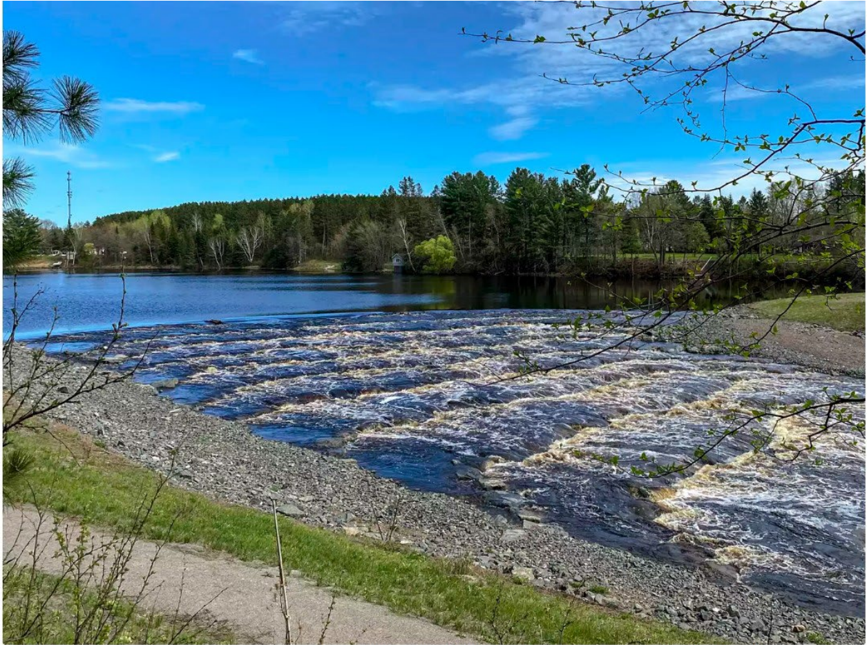
The Willow River dam in Pine County, near its confluence with the Kettle River, failed in 2016 and was replaced with rock arch rapids, completed in 2022. 🟡 Courtesy of Minnesota Department of Natural Resources
