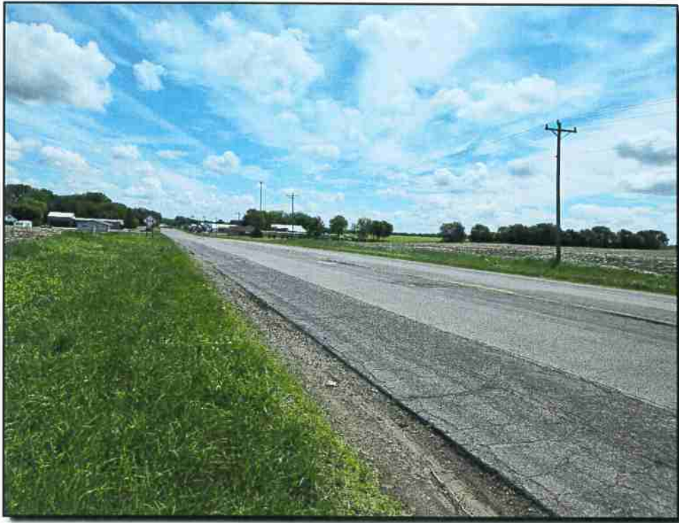
Photograph showing Lake Avenue, taken near the center of south boundary of the north parcel of the subject property, facing east.
